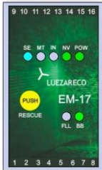
Lift on the floor with doors closed
